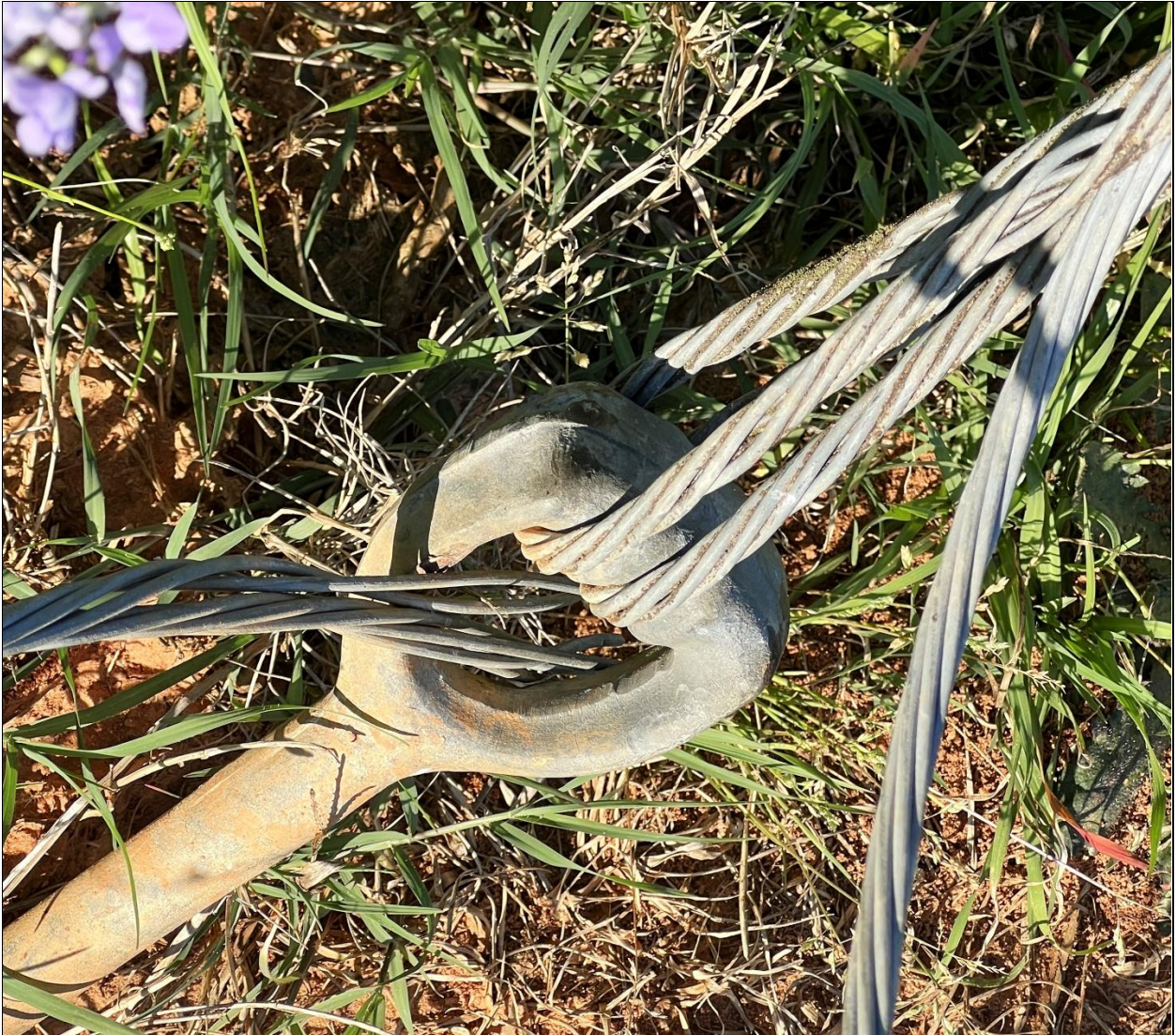
Figure 2 guy anchor with forged saddle end
